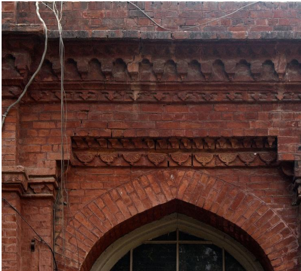
Figure 12. Details of moulded brick decoration on the façade of the southern wing Source: Photograph October 20, 2024
