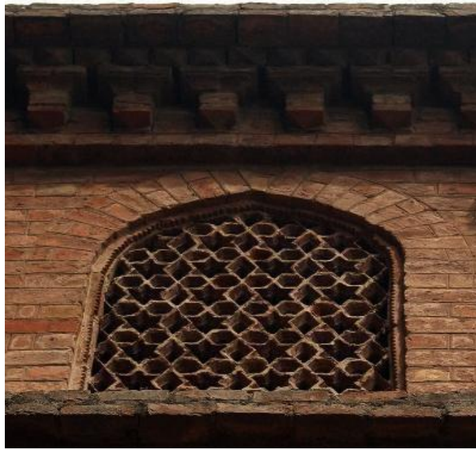
Figure 16. Terracotta Lattice or Jāli work on the building at the back of the southern wing type 4 Source: Photograph October 20, 2024
