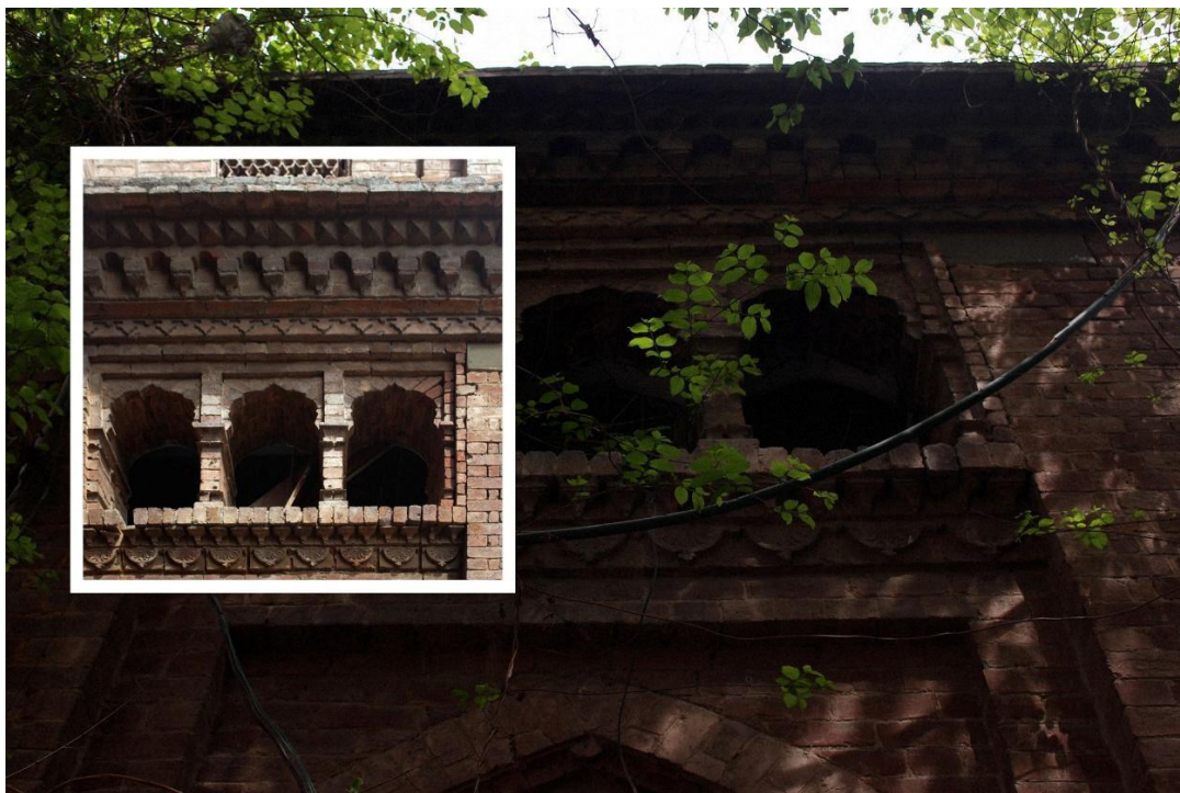
Figure 17. Multifoil arched windows for light and ventilation on the building at the back of the southern wing
