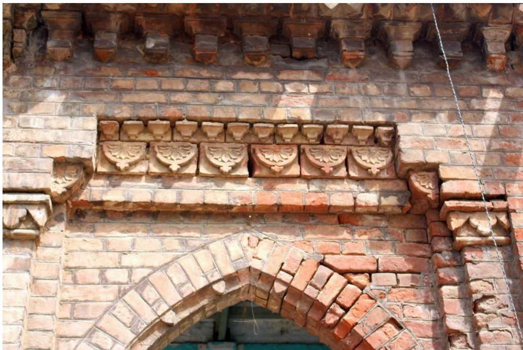
Figure 15. Close-up of moulded brick design details at the building's backside the southern wing
