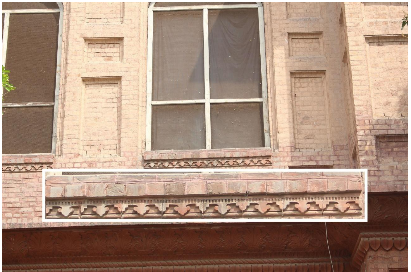
Figure 9. Details of moulded brick decoration under the sill on northern wing Source: Photograph October 20, 2024
