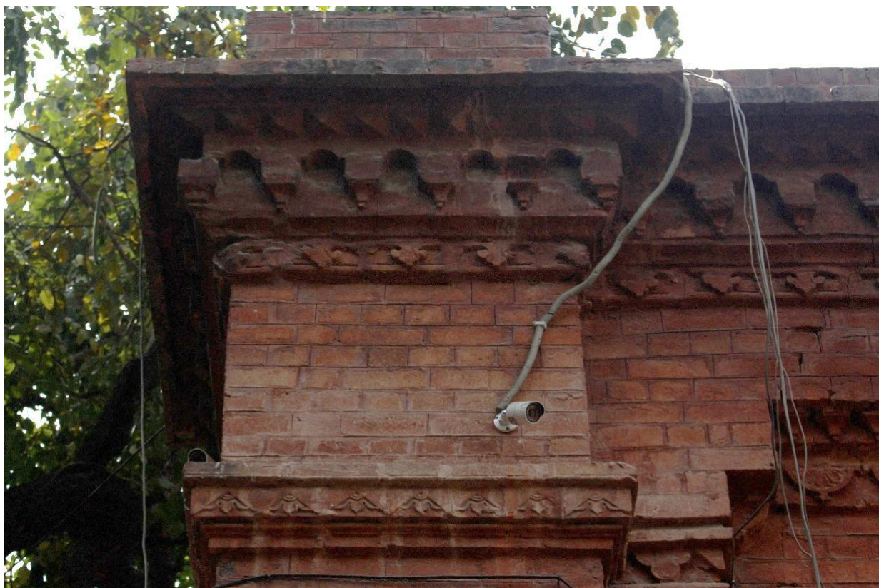
Figure 11. Details of moulded brick decoration on the cornice of the southern wing Source: Photograph October 20, 2024
