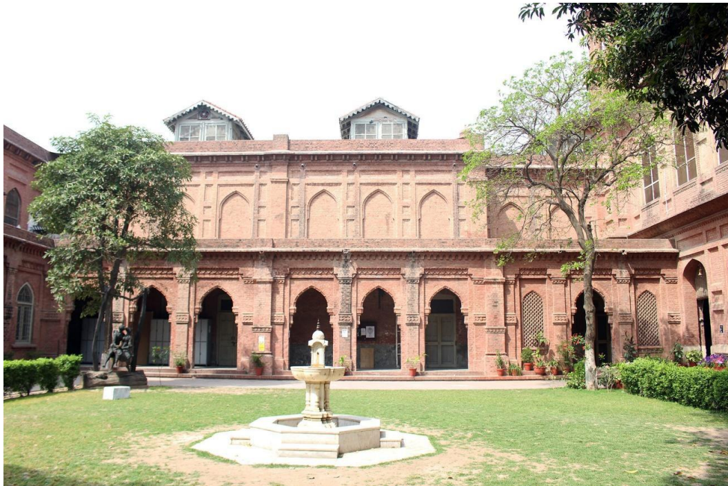
Figure 1. View of the northern wing facing courtyard Source: Photograph October 20, 2024
