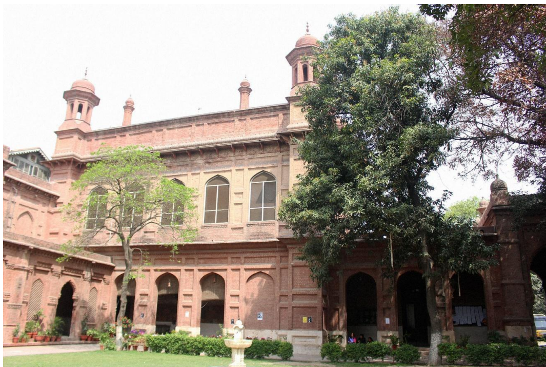
Figure 2. View of the western wing facing courtyard Source: Photograph October 20, 2024
