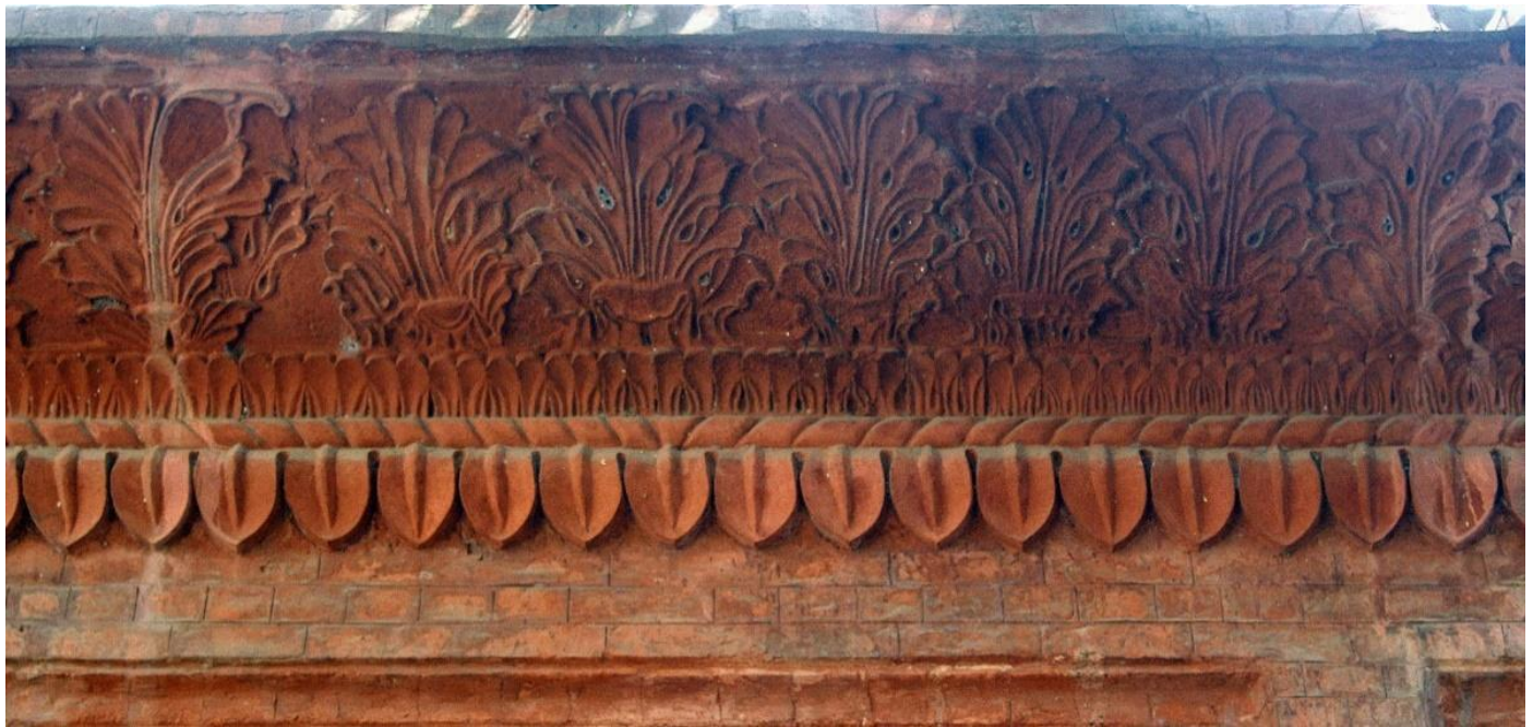
Figure 8. Details of moulded brick designs on the frieze inside the northern wing Source: Photograph October 20, 2024
