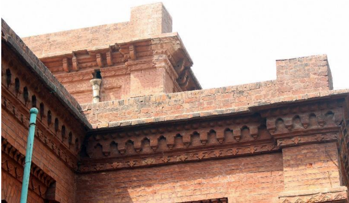
Figure 10. Details of moulded brick decoration on western and southern wings Source: Photograph October 20, 2024
